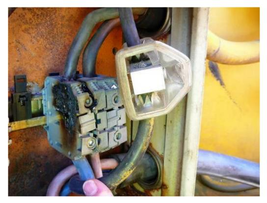
Previous fire damage, and a "watertight" connection jury rigged with a Tupperware type container
