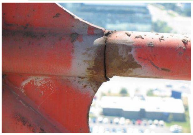
A crack completely through a critical structural member, could reduce crane capacity significantly
